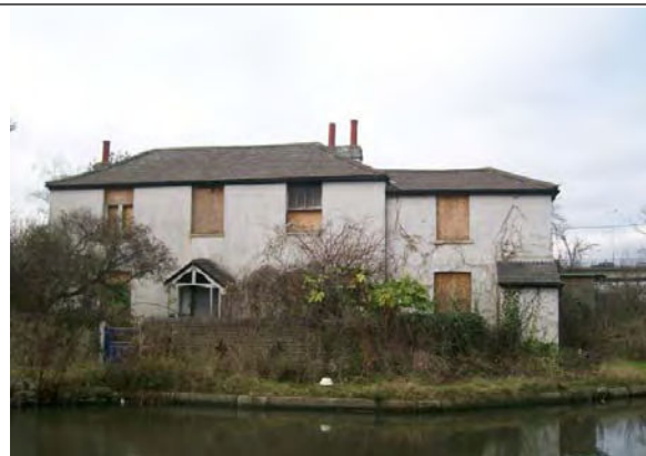
Front elevation from the Canal
