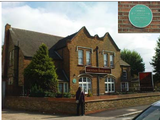
Elevation fronting Church Road
