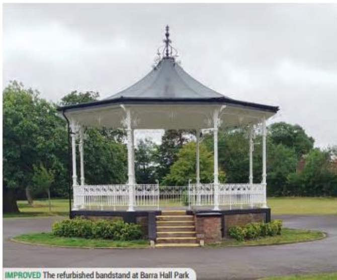
IMPROVED The refurbished bandstand at Barra Hall Park
