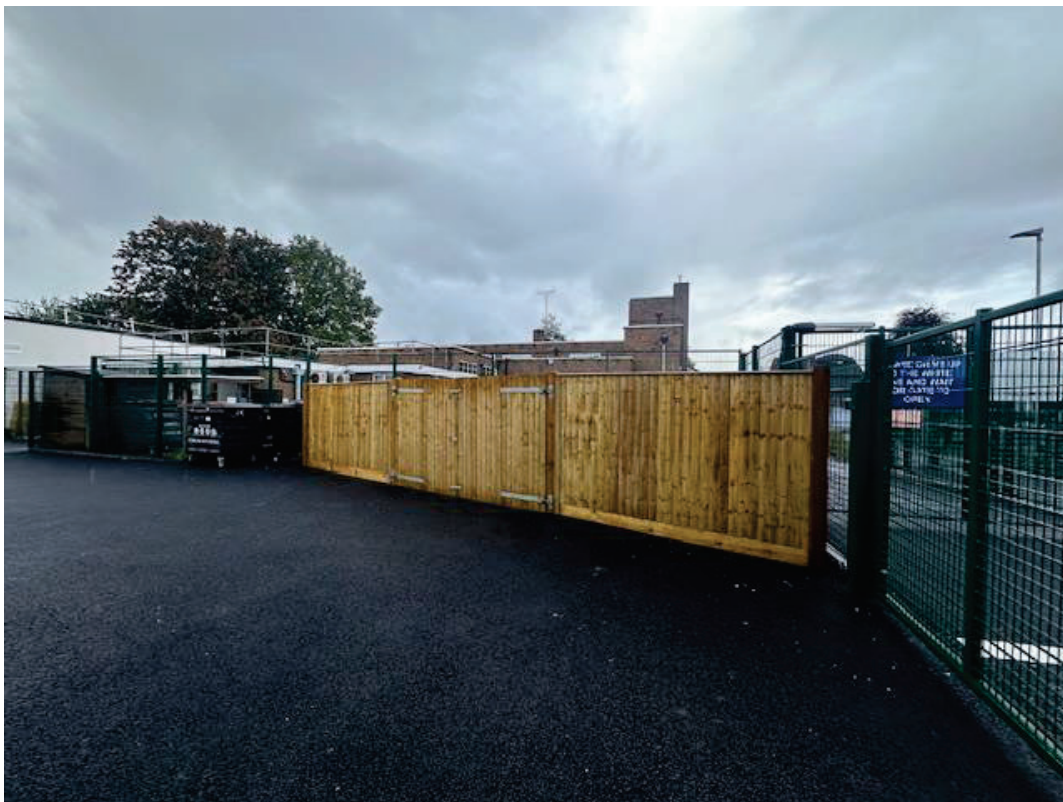
Figure 2: Photograph of the Application Site – Bin Storage Area
