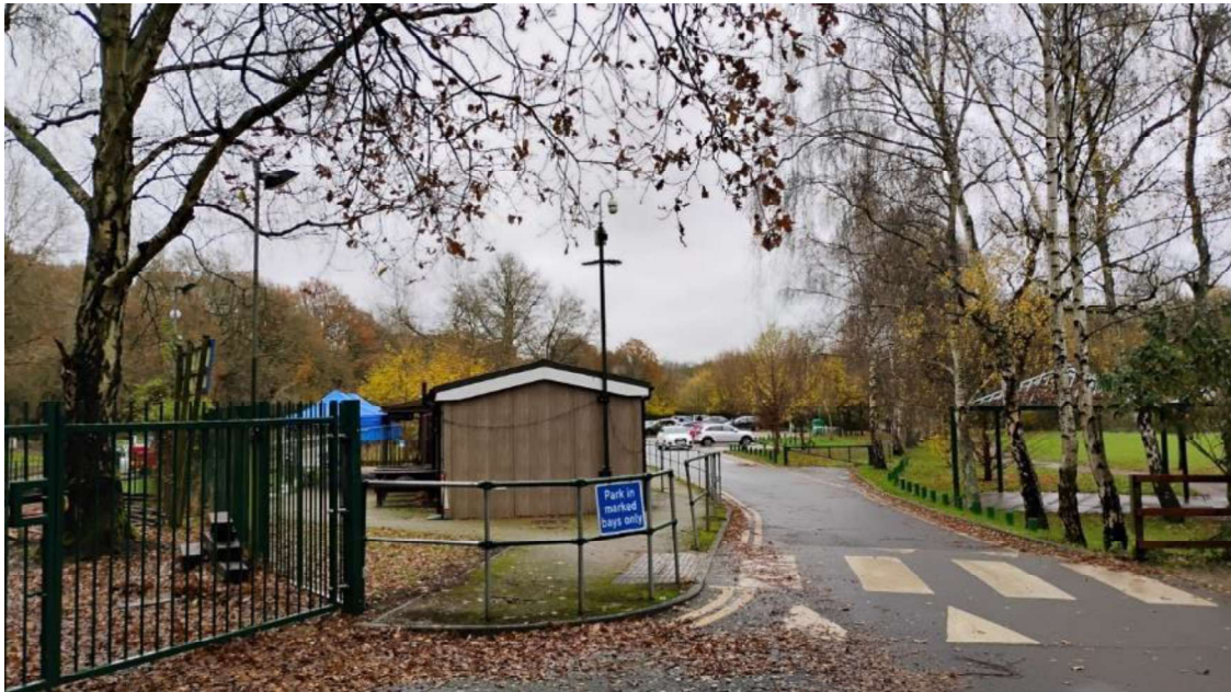
Figure 10: Existing side elevation of Willow Lawn toilet block as viewed from main vehicle entrance.
