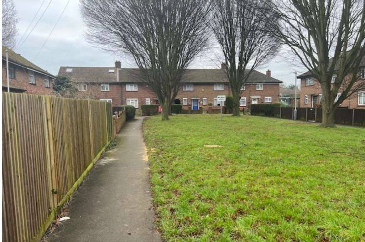
Figure 2: Street View Image of the Application Property (furthest terrace to the left)
