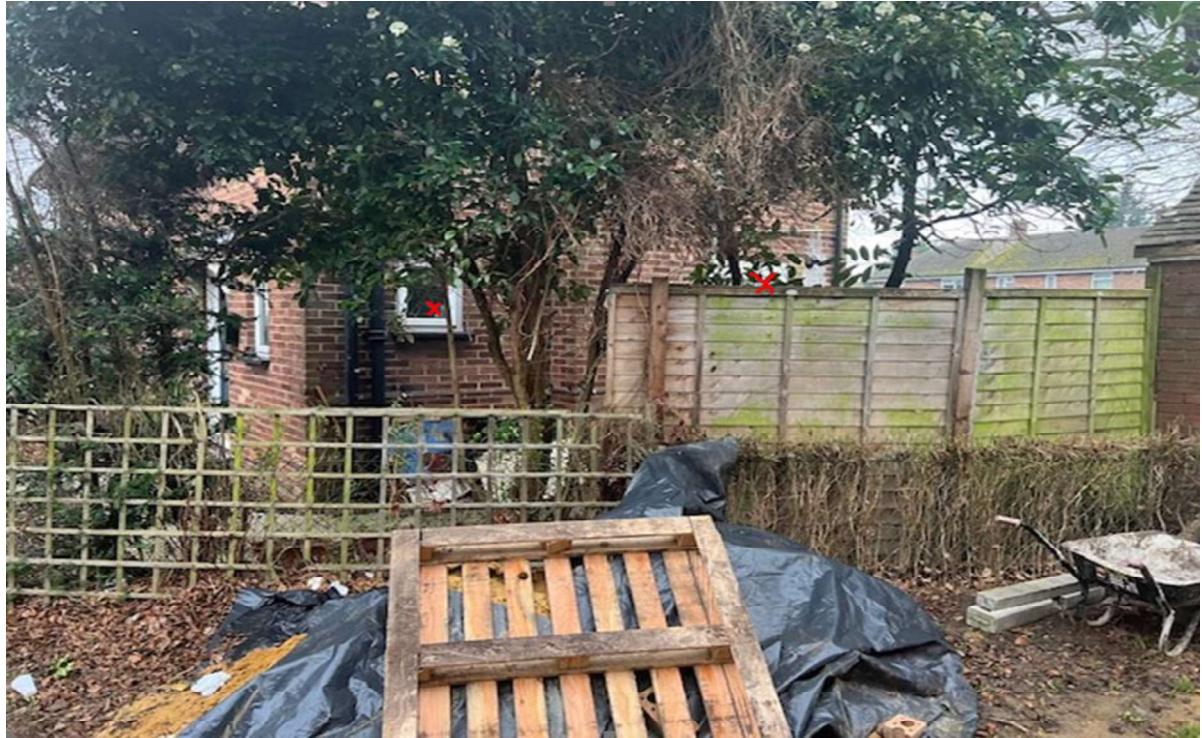
Figure 5: 11 Oak Avenue ground Floor side windows
