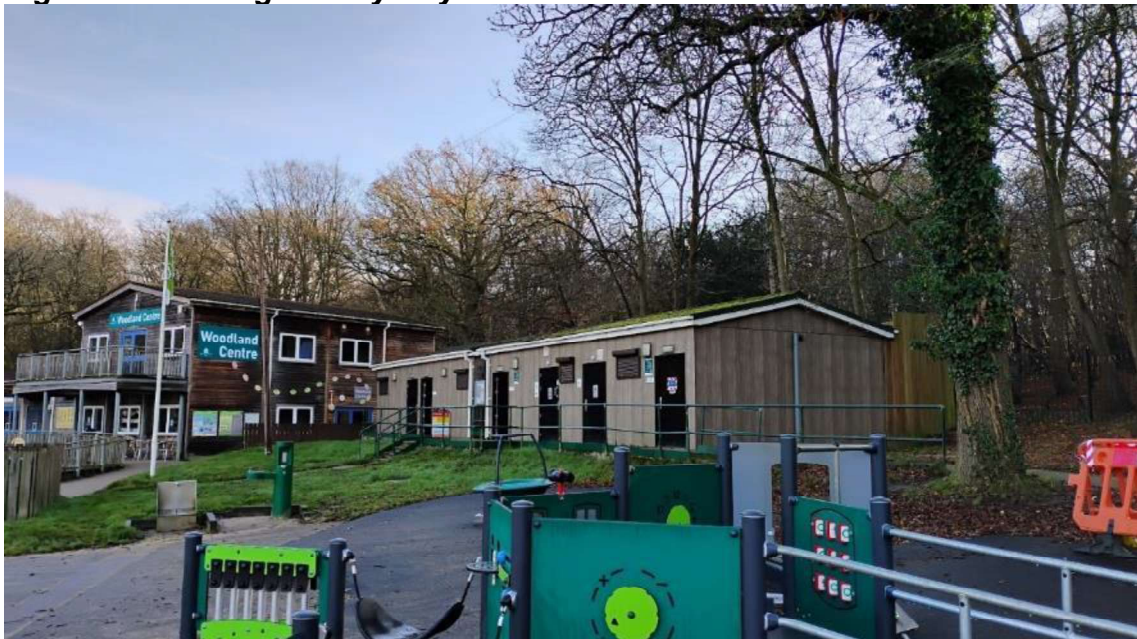
Figure 5: Existing Woody Bay toilet block.
