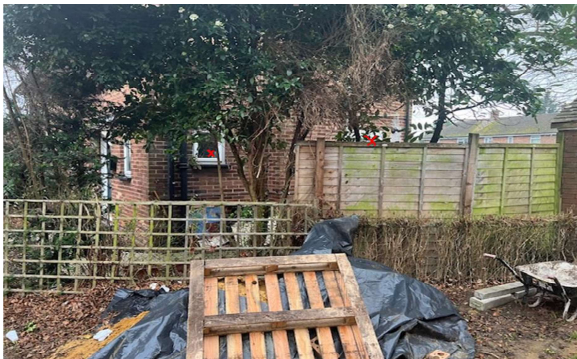
Figure 5: 11 Oak Avenue ground Floor side windows
