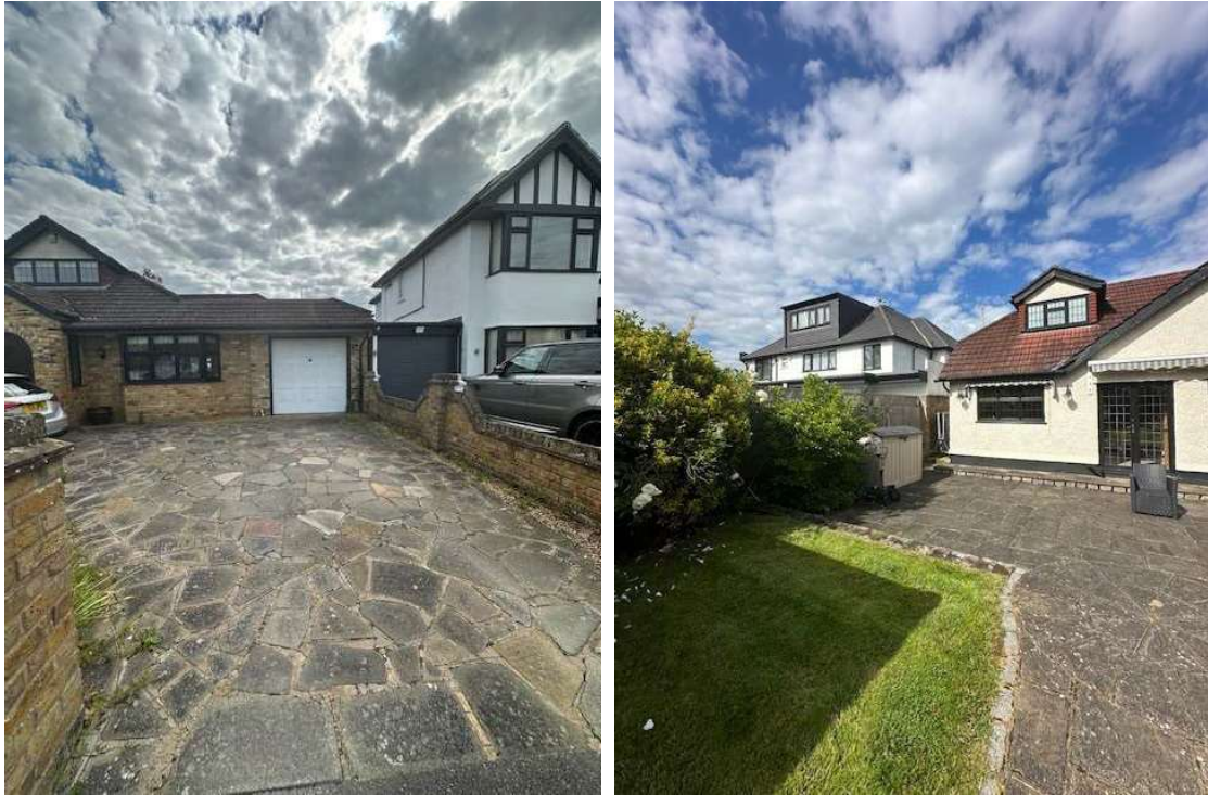
Figures 6-7: Photographs of the boundary with 43 Parkfield Road at the front and rear of the Application Property
