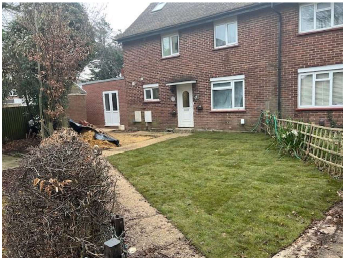
Figure 3: Front Elevation of the Property
