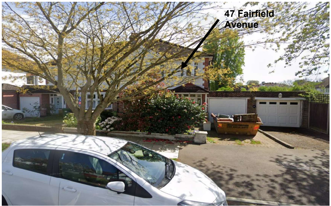
Figure 2: Street View Image of the Application Property.
