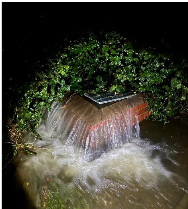
Figure 5-4: Photograph of the surface water sewer in Bessingby Park surcharging on the 23 September 2024. Image credit: Whitby Road resident.
