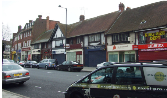
Fig 6.1: Early 20 th century shops on the High Street (Nos 56-62)
