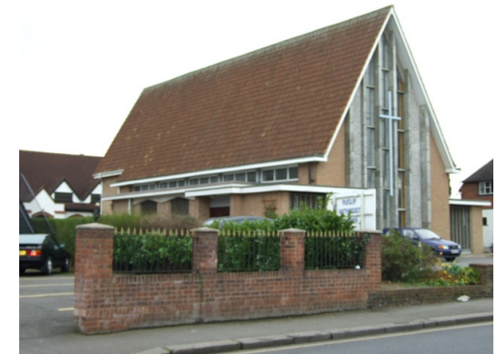
Fig 7.21: Ruislip Methodist Church, Ickenham Road
