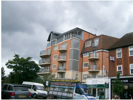
Fig 7.22: The Thomas Moore building, Ickenham Road
