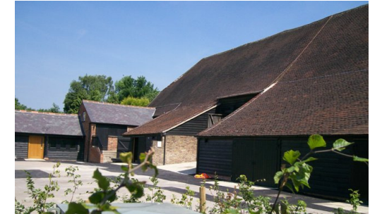
Fig 5.22: Clay tiled roof (the Great Barn)
