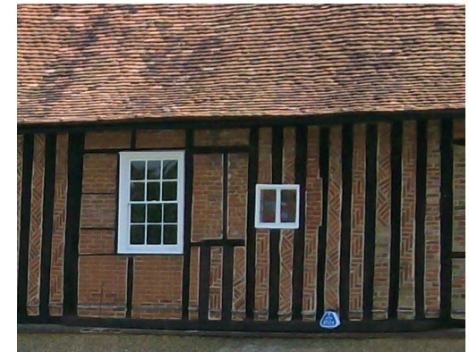
Fig 5.19: Brick noggin- Manor Farm
