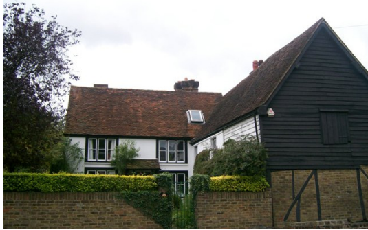
Fig 5.15: The Mill House, Bury Street (Grade II)
