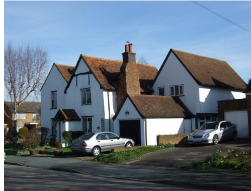
Fig 7.11: Laurel Cottage, Primrose Cottage and Tudor Cottage, Wood Lane
