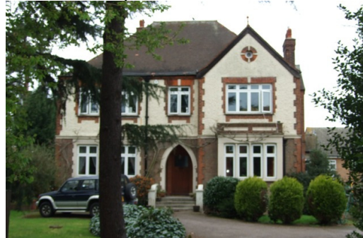
Fig 7.20: No 28 Ickenham Road
