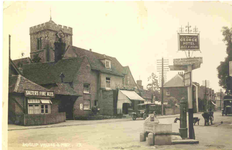
Fig 5.27 Original position of the pump
