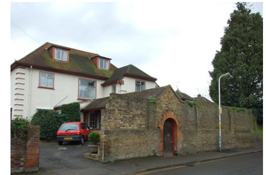
Fig 7.1: Walls fronting No 9 Sharps Lane
