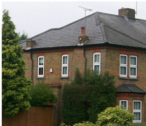
Fig 5.21: Semi-detached houses on Bury Street in stock brick with red brick detailing
