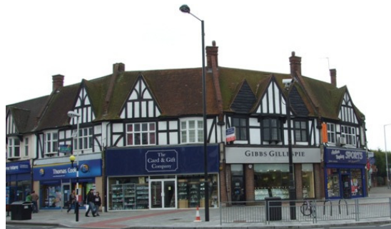
Fig 6.2: Nos 92-96 High Street- decorative timber framing, bold gables and distinctive tall chimney stacks
