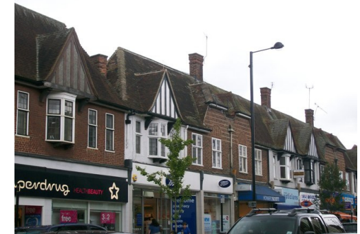
Fig 6.3: Nos 110-114 High Street- mock timber framing with oriel windows
