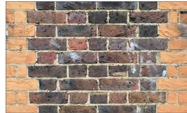
Brown and red brick with lime mortar
