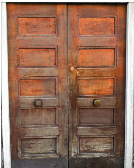
Art Deco five panel door with original door furniture
