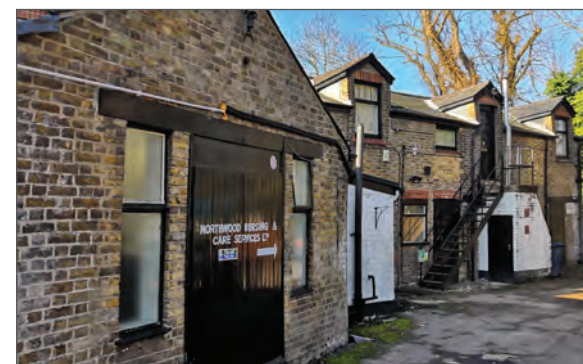
Outbuilding, rear of Green Lane
