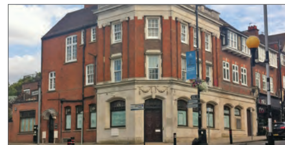
Former NatWest Bank, Green Lane
