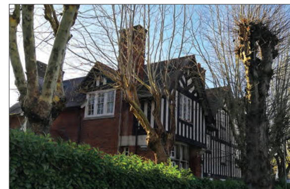
Police Station, 2 Murray Road, north elevation
