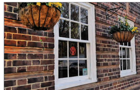
Six over six timber sash windows
