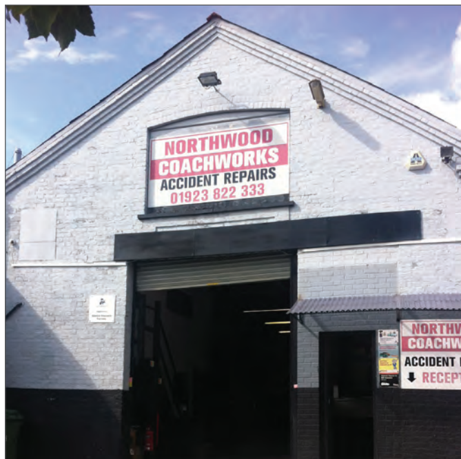
Railway sheds behind Station Approach
