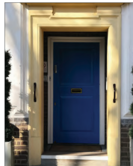
Original recessed door and stone door surround
