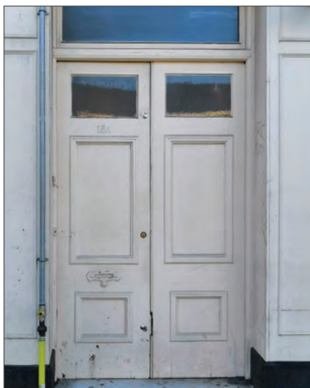
Timber double door, door light
