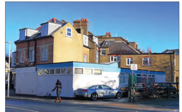
Rear of 3-27 Maxwell Road shops
