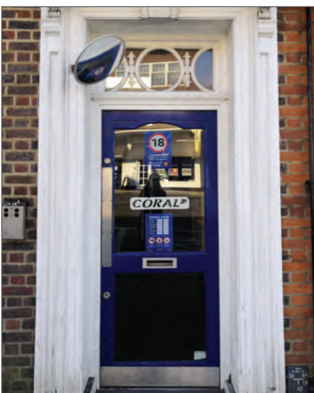
Neo-Georgian painted timber door surround
