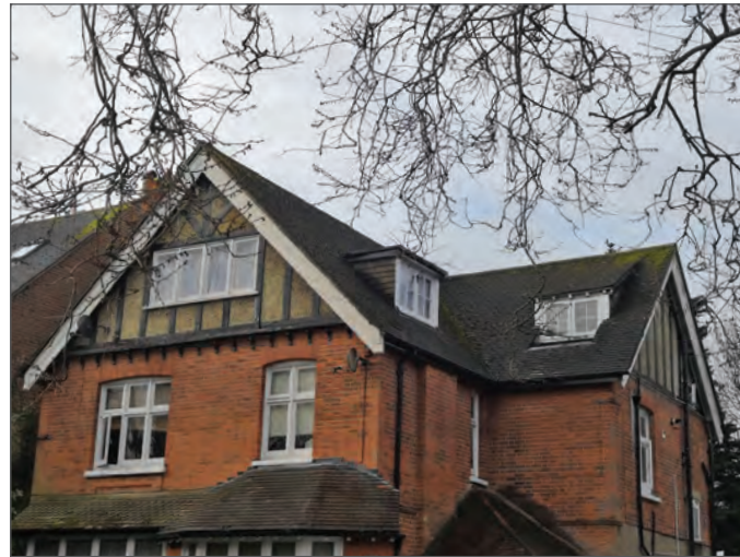
Gable roofs with half-timbered gable
