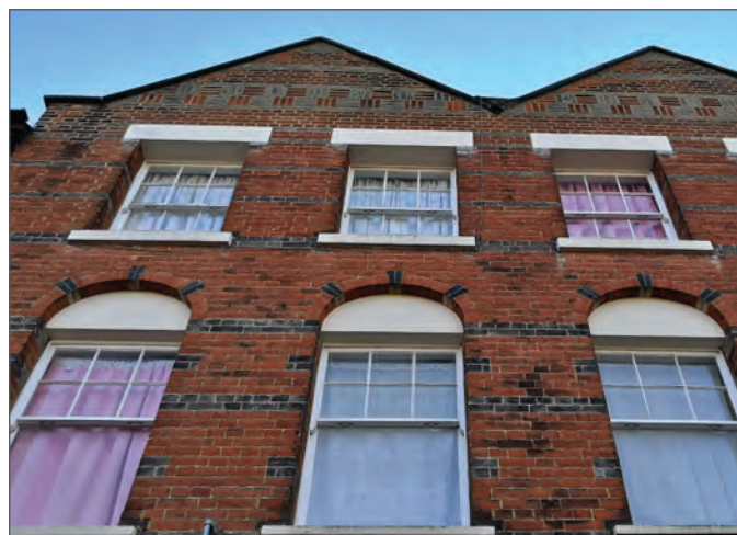
Six over one timber sash windows with horns
