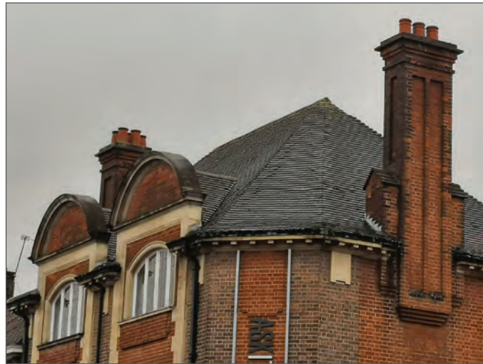
Hipped roof with decorative brick stack
