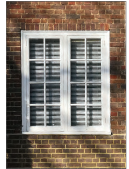
Small paned timber casement
