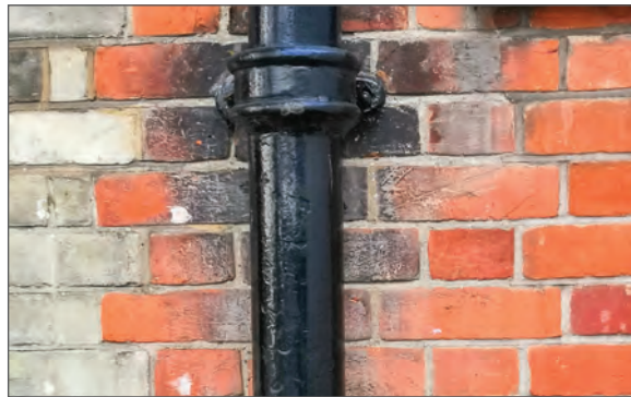
Cast iron downpipe
