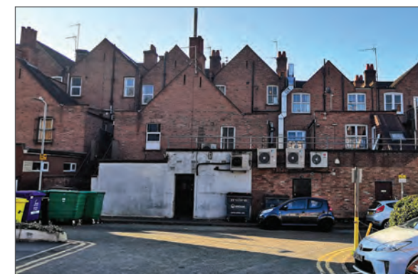
Rear of 39-51 Green Lane
