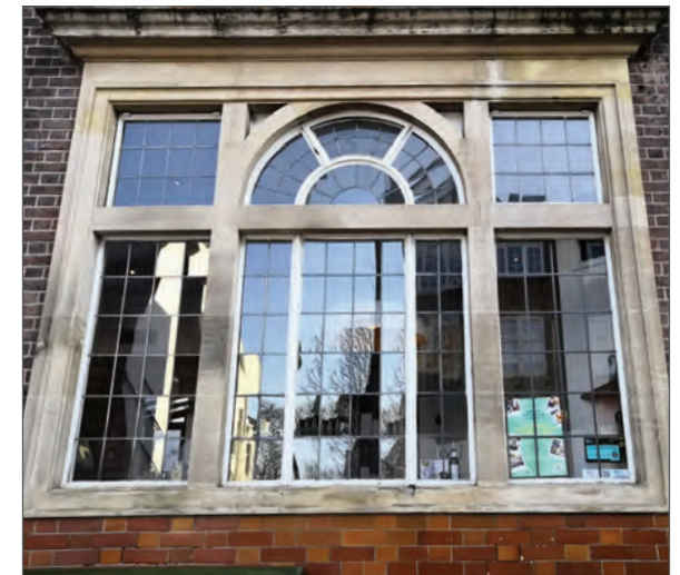
Serliana transom and mullion window with leaded lights
