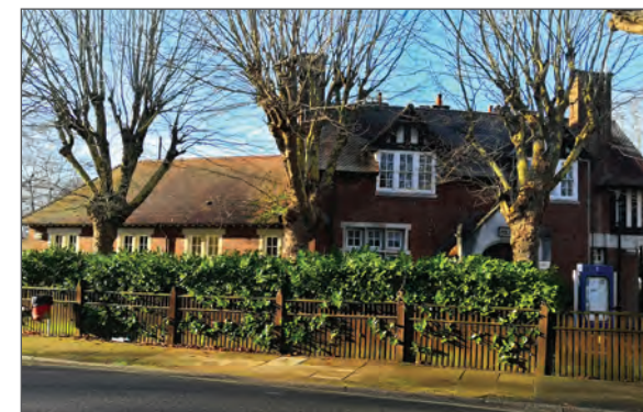
Police Station, 2 Murray Road, east elevation
