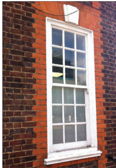
Nine over nine timber sash with horns
