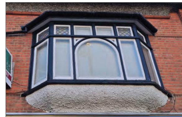
Ogee and dormer windows
