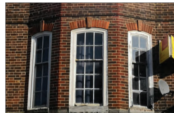
Bay window with small paned sashes
