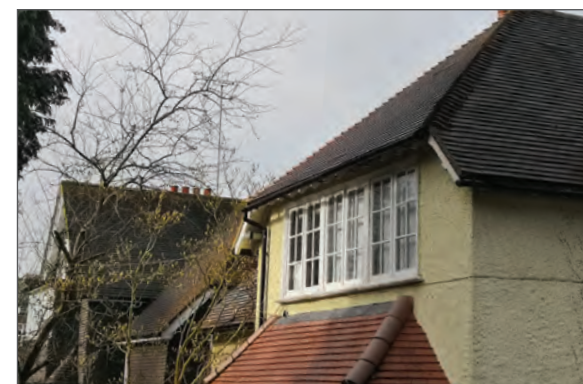
Three quarter hipped roof
