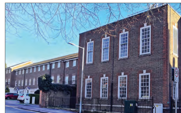
Telephone exchange, Dene Road
