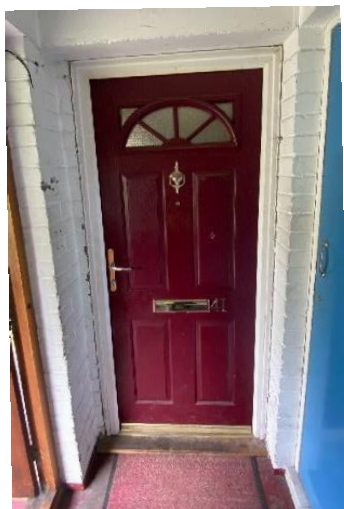
Before photo of a front entrance door
