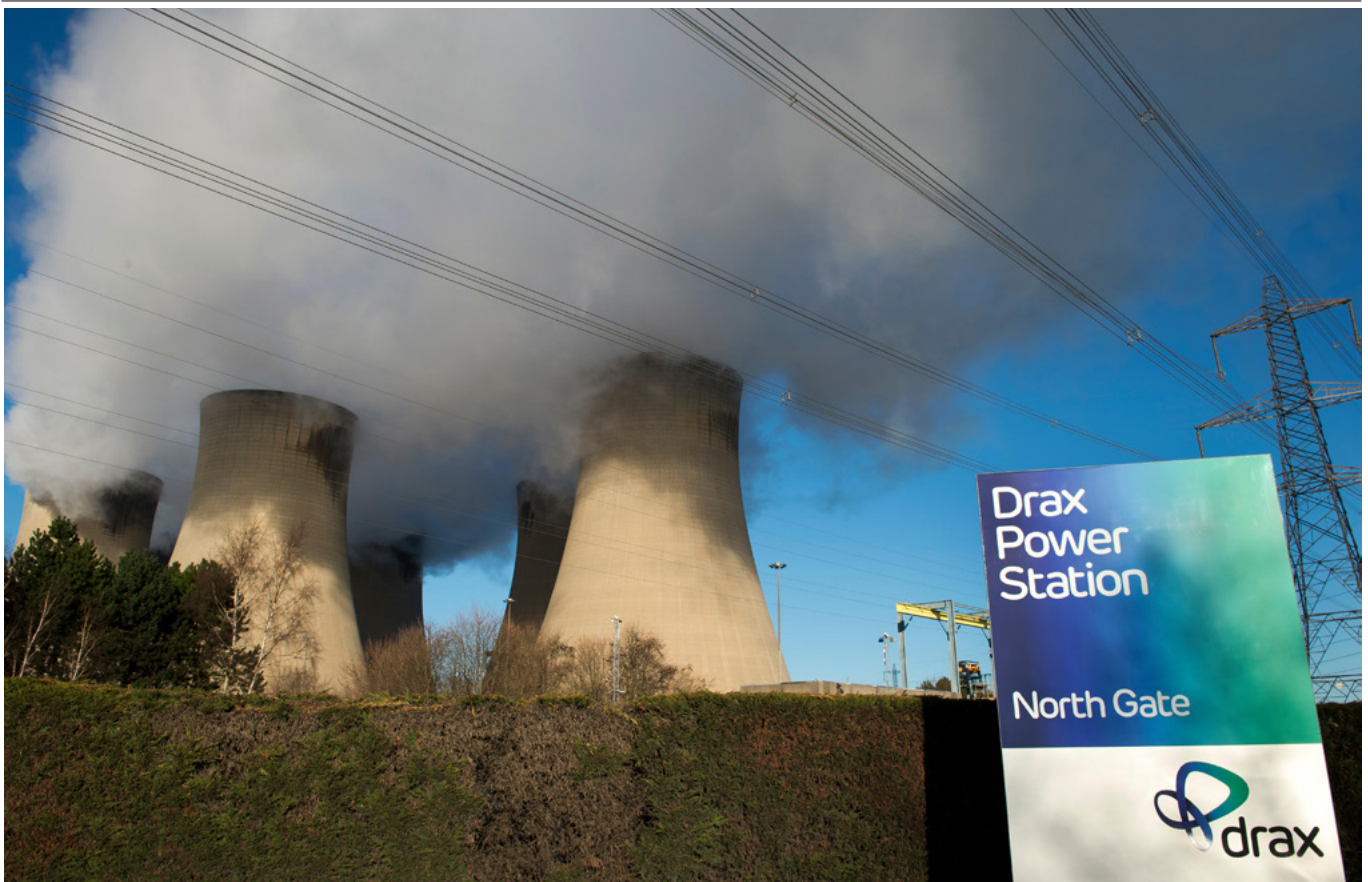
Cooling towers at Drax Power Station near Selby, North Yorkshire.
