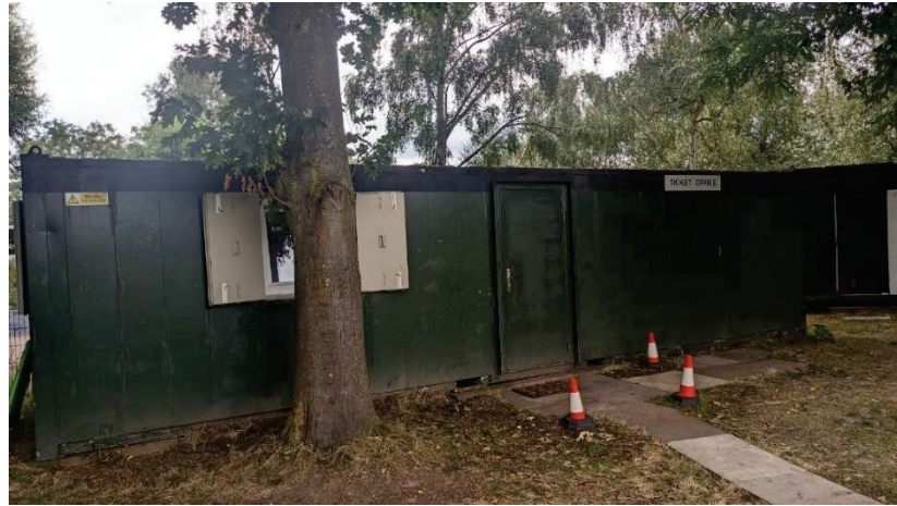
Figure 4: Existing Container Location in the context of Roxbourne Park
