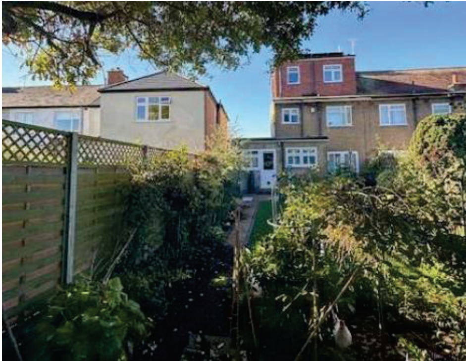
Figure 4: Extension as built taken from rear garden of 102 Exmouth Road
