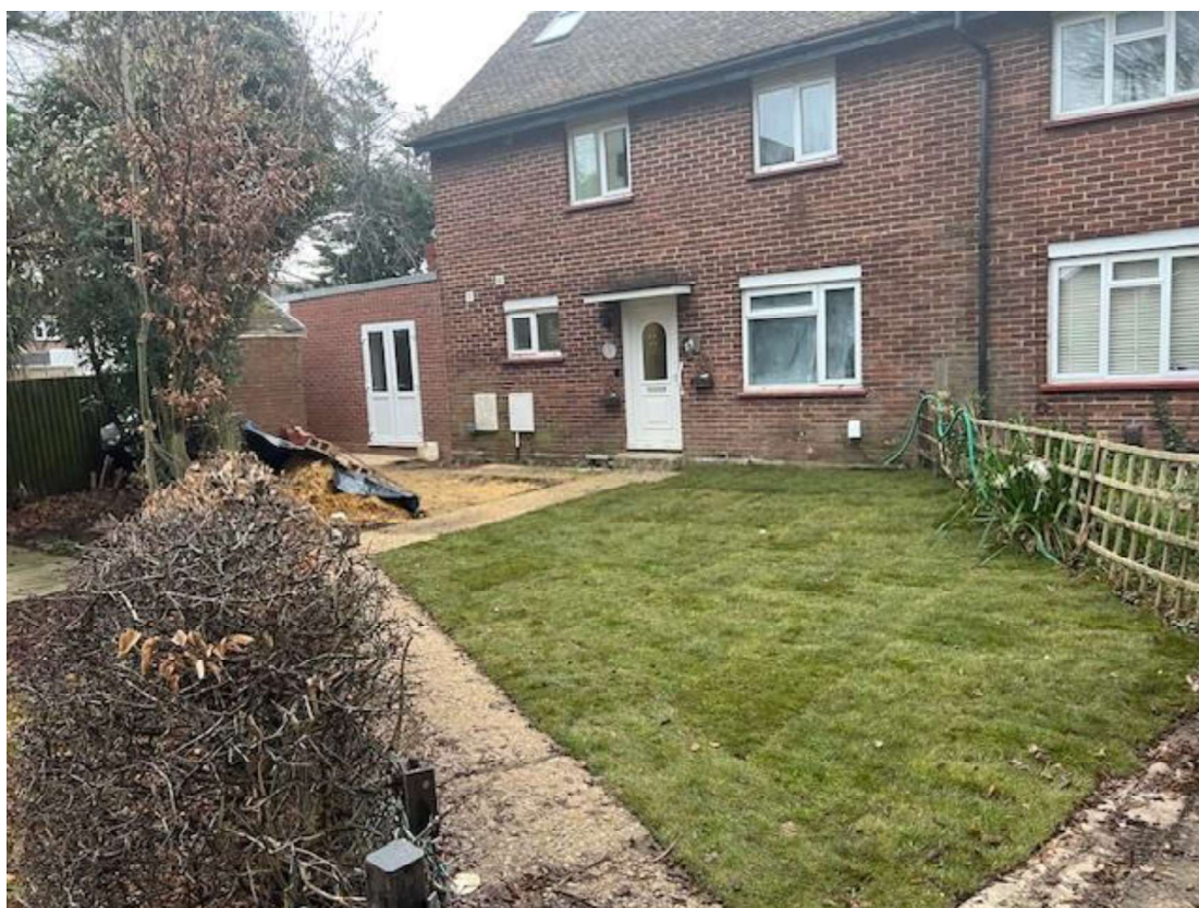
Figure 3: Front Elevation of the Property
