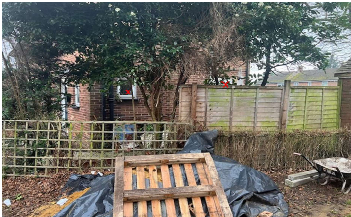
Figure 5: 11 Oak Avenue ground Floor side windows
