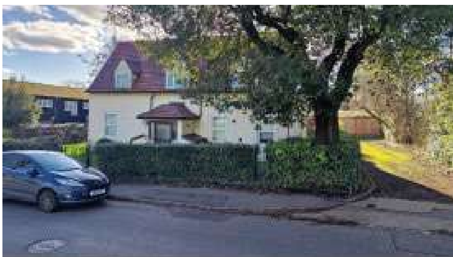
Figure 4: Rear elevation of the existing property
