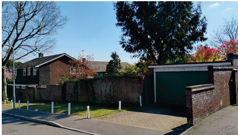
Figure 4: Rear elevation of the property.
